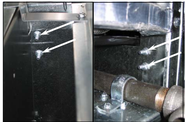
Figure 5. Insert bolts, but do not tighten.
